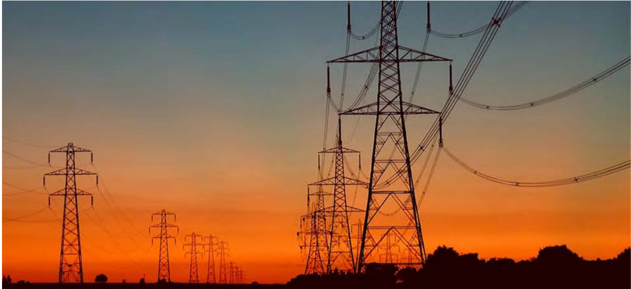
Figure 15.1 The current we draw into our houses is an alternating current (ac). Power lines transmit ac to our neighborhoods, where local power stations and transformers distribute it to our homes. In this chapter, we discuss how a transformer works and how it allows us to transmit power at very high voltages and minimal heating losses across the lines.
