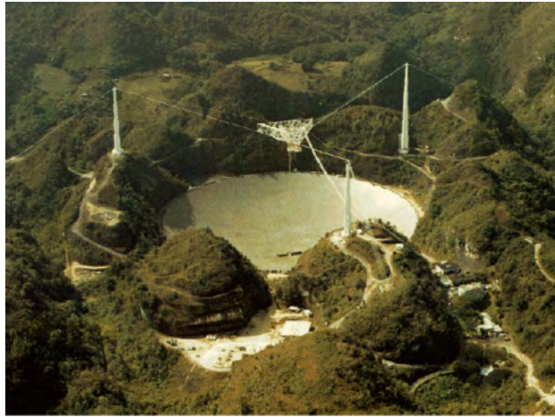
Figure 6.22 Largest Radio and Radar Dish. The Arecibo Observatory, with its 1000-foot radio dish-filling valley in Puerto Rico, is part of the National Astronomy and Ionosphere Center, operated by SRI International, USRA, and UMET under a cooperative agreement with the National Science Foundation. (credit: National Astronomy and Ionosphere Center, Cornell U., NSF)
