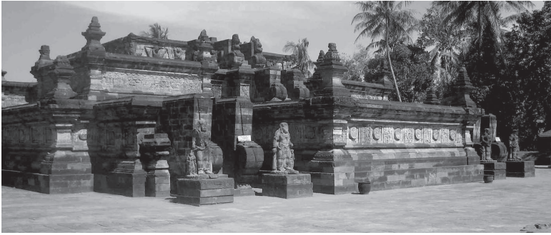
Fig. 7.40. Main Temple in the third courtyard, view from northwest
