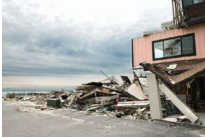
Figure 1.5 A Photo of Galveston Island after Hurricane Ike
