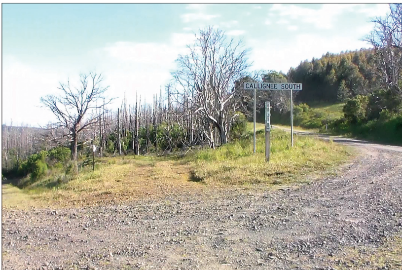
Figure 12.6: Example of rural roads.
