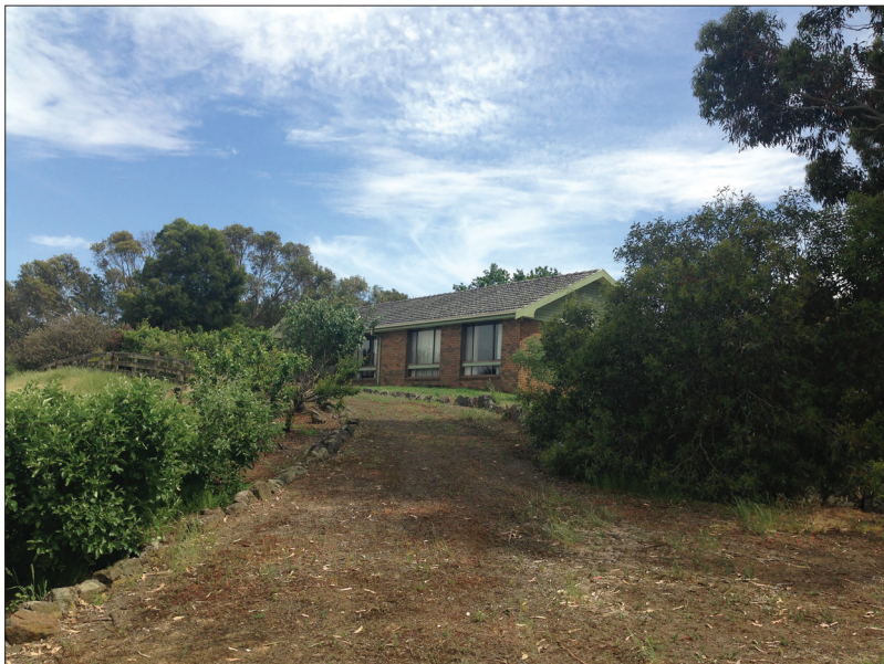
Figure 12.2: A regional home in Victoria.
