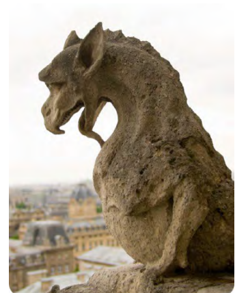
Figure 44: This chimera at Notre Dame Cathedral in Paris exhibits damage from acid rain.
