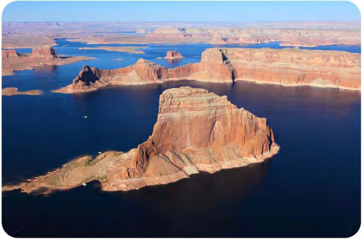
Figure 166: Glen Canyon Dam in Arizona created Lake Powell. The dam was controversial because it flooded Glen Canyon, a beautiful desert canyon.
