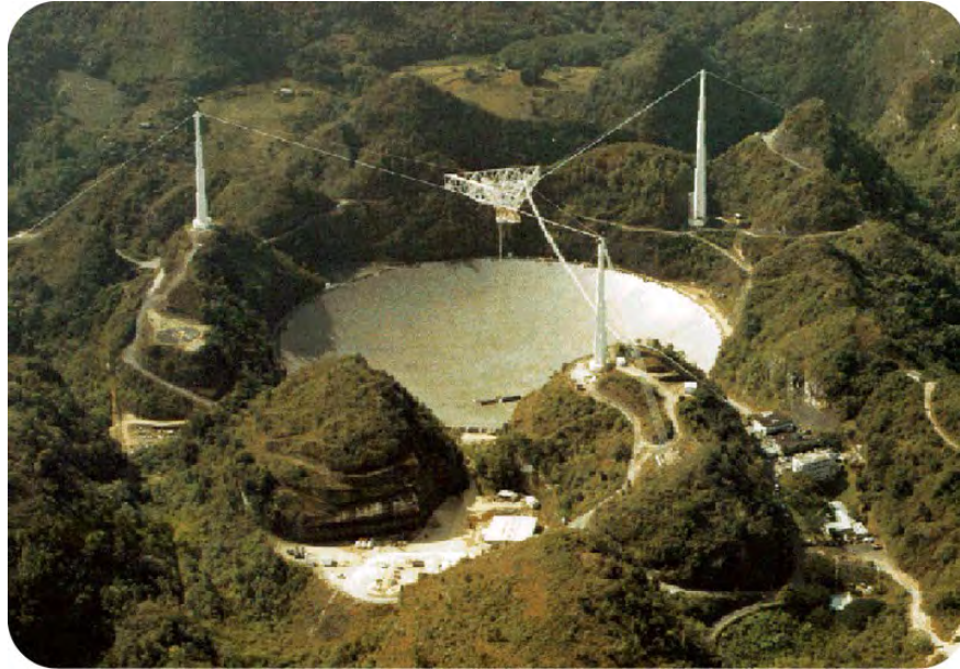
Figure 232: The radio telescope at the Arecibo Observatory has a diameter of 305 m.
