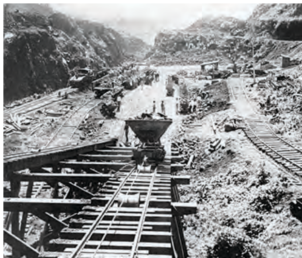
Figure 22.15 Recurring landslides made the excavation of the Culebra Cut one of the most technically challenging elements in the construction of the Panama Canal.
