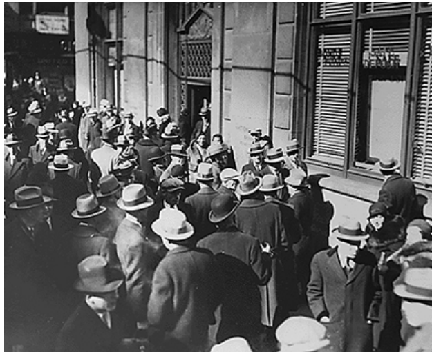
Figure 25.5 As the financial markets collapsed, hurting the banks that had gambled with their holdings, people began to fear that the money they had in the bank would be lost. This began bank runs across the country, a period of still more panic, where people pulled their money out of banks to keep it hidden at home.
