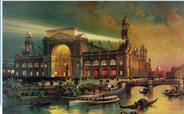
Figure 18.1 The Electrical Building, constructed in 1892 for the World's Columbian Exposition, included displays from General Electric and Westinghouse, and introduced the American public to alternating current and neon lights. The Chicago World's Fair, as the universal exposition was more commonly known, featured architecture, inventions, and design, serving as both a showcase for and an influence on the country's optimism about the Industrial Age.
