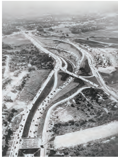
Figure 28.13 In the late 1940s, a network of newly constructed highways connected suburban Long Island with Manhattan. The nation's new road network also served a military purpose; interstate highways made it easier to deploy troops in the event of a national emergency.
