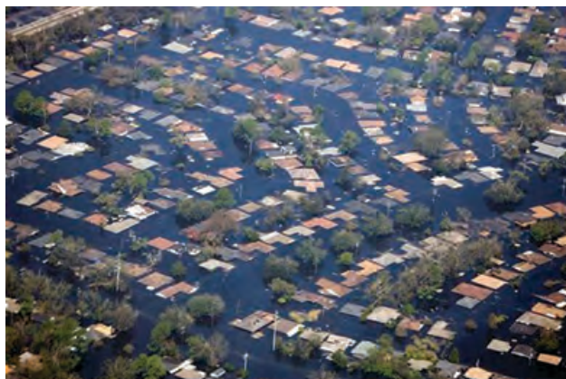
Figure 32.10 Large portions of the city of New Orleans were flooded during Hurricane Katrina. Although most of the city's population managed to evacuate in time, its poorest residents were left behind.
