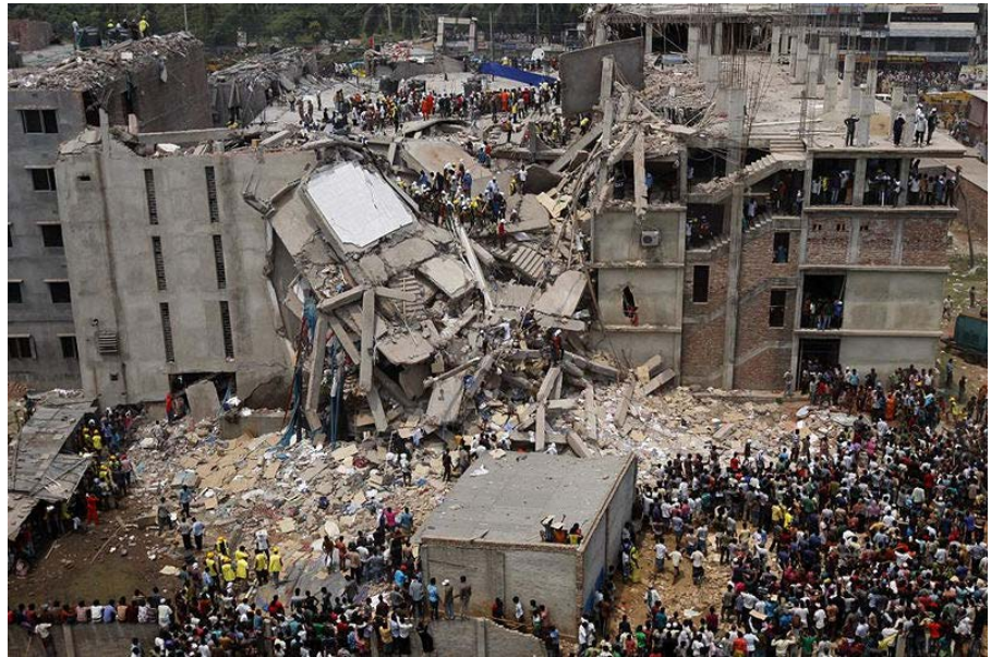
Figure 7.6. The Rana Plaza (Savar) Factory Collapse, Bangladesh
