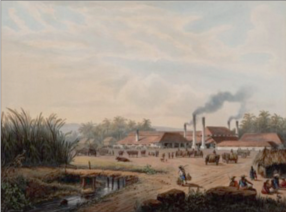
Figure 8: Mid-nineteenth-century industrialisation: there is no extant painting or photograph of the Wonopringgo sugar factory in the mid-century decades. This contemporary view of the Pangka factory further along the north coast of Central Java provides some indication of what Wonopringgo must have been like.
