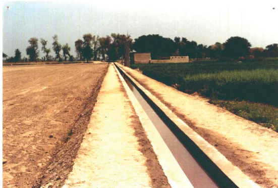
Figure 8: Earthen watercourse improvement.
