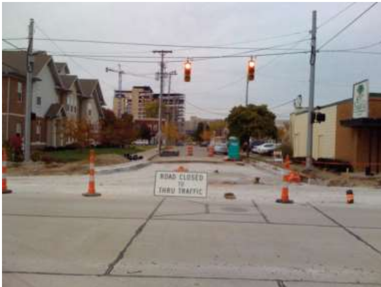
Figure 7.1 A Typical Construction Site
