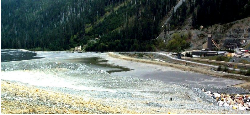
Figure 20.12 The tailings pond at the Myra Falls Mine on Vancouver Island. The dry rock in the middle of the image is waste rock. The structure on the right is the headframe for the mine shaft. Myra Creek flows between the tailings pond and the headframe. [SE]
