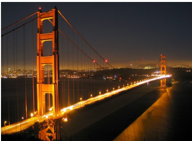
q / The Golden Gate Bridge's roadway is held up by the tension in the vertical cables.
