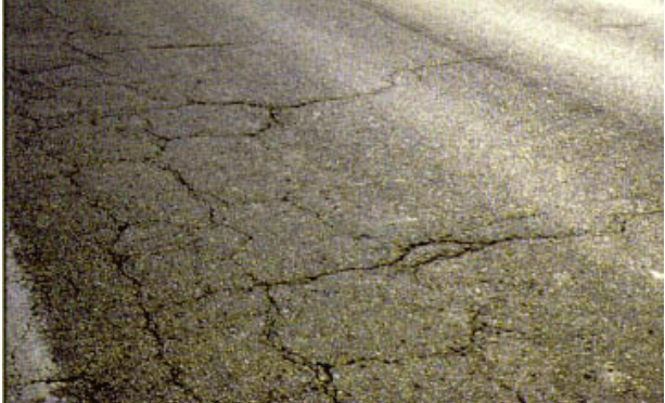
Figure 3.9 - Block Cracking in Asphalt Pavements
