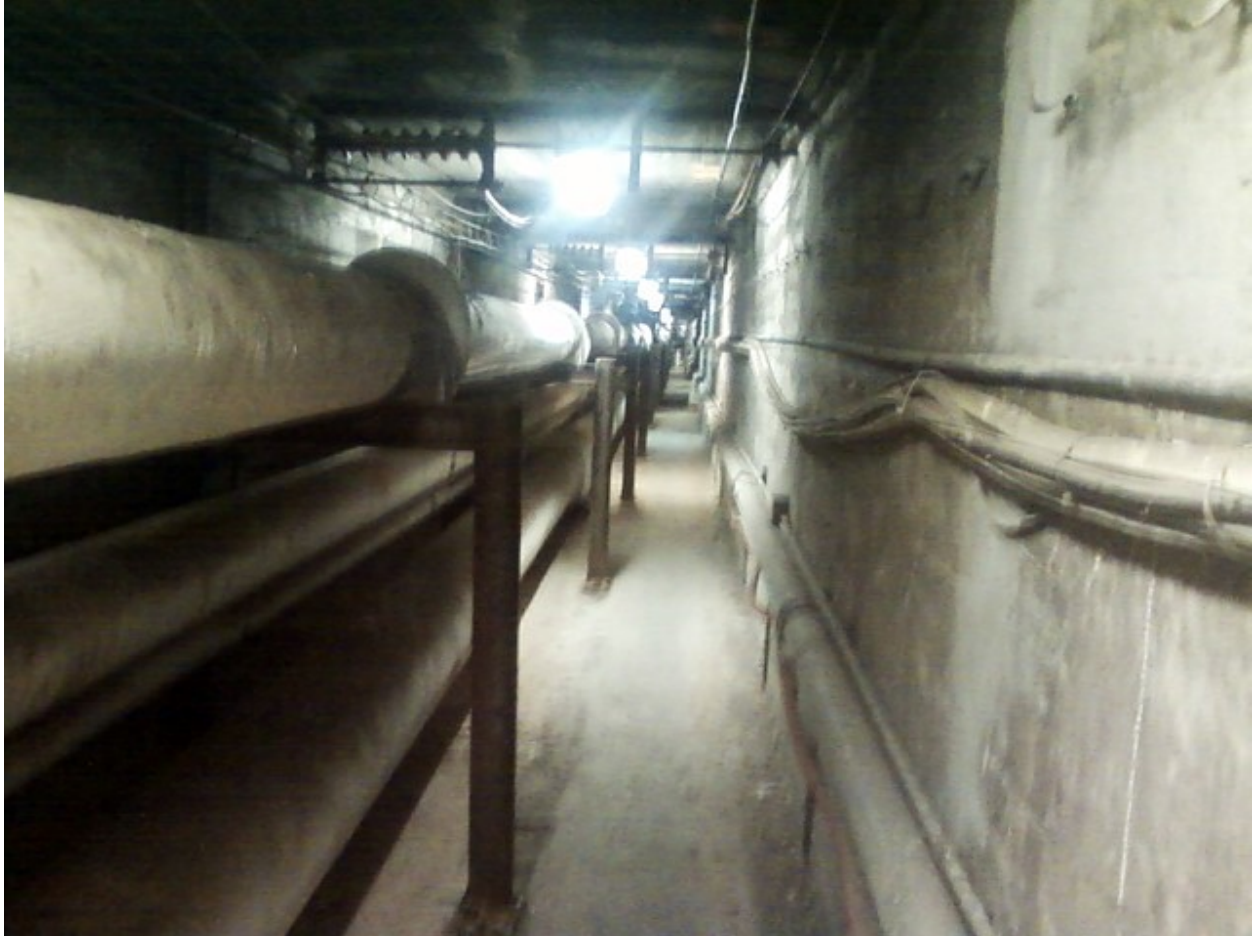
Figure 16.8 - Illustration of a Small Utilidor on a University Campus
