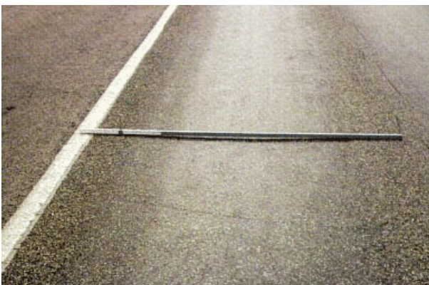
Figure 3.13 - Rutting and Depressions in Asphalt Pavements
