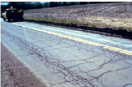
Figure 3.8 - Alligator Cracking in Asphalt Pavements
