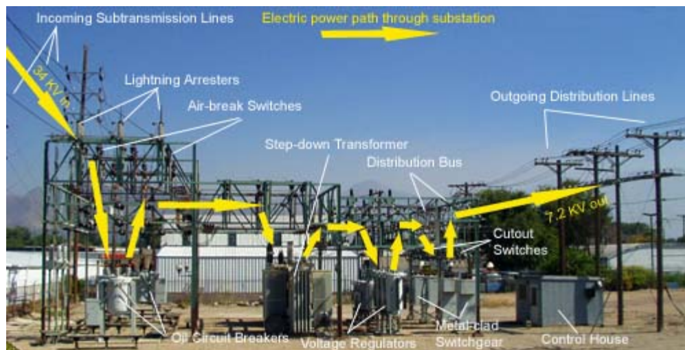
Figure 15.8 -Components of a Typical Substation
