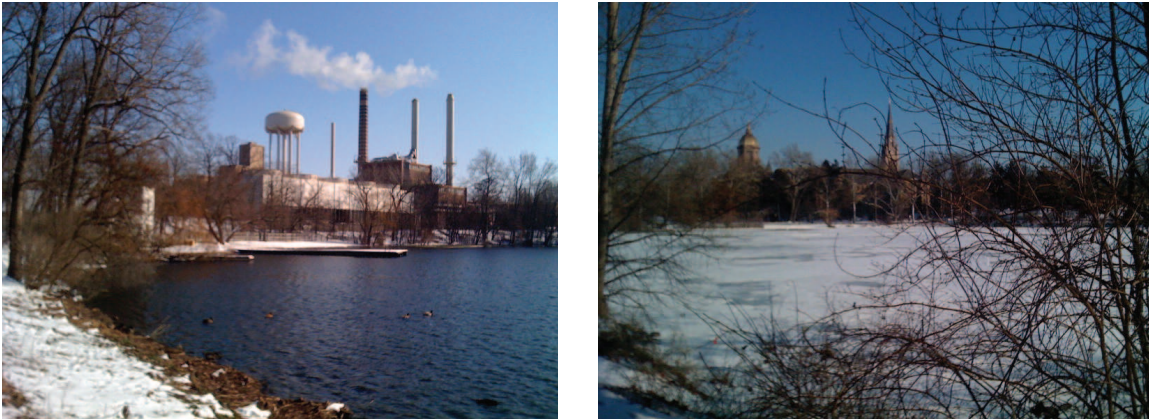
Figure 6.21: St. Joseph's Lake (left) and St. Mary's Lake (right) on the University of Notre Dame campus, 14 February 2010, demonstrating the effect of exchanging heat with the condenser of the Notre Dame power plant near St. Joseph's Lake.
