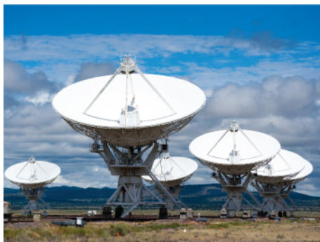
Figure 2.86 Energy reflects off of the parabolic reflector and is collected at the focal point. (credit: modification of CGP Grey, Wikimedia Commons)
